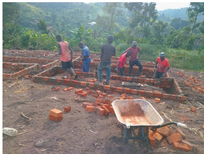
Garden beds being constructed. Clay bricks are made locally.
